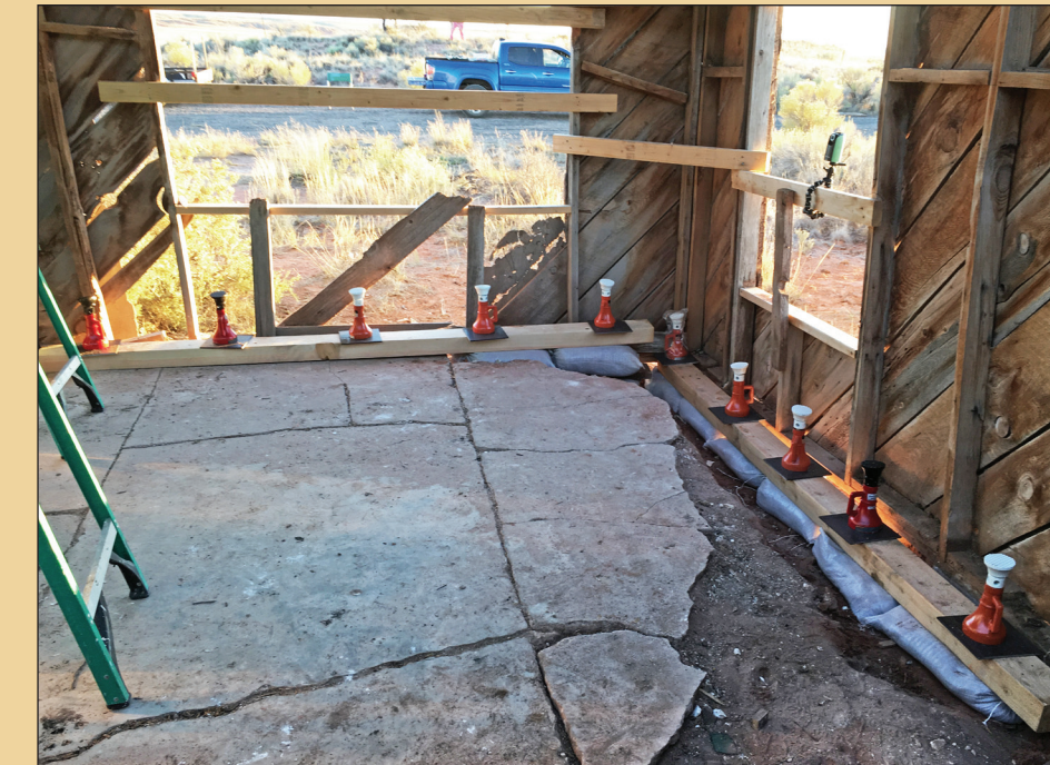
Sandbags and timbers created a stable platform for raising walls.
