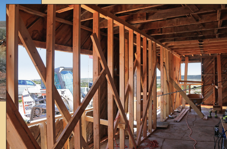
Once correct elevation was obtained, shear walls were built thirty inches inside existing exterior walls to hold the repositioned building in place.
