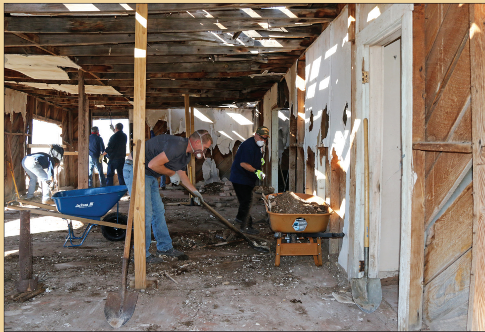
Clearing the debris and removing old sheetrock took a full day.
